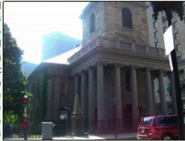
King's Chapel West Elevation. (Photo courtesy of Goody & Clancy)
