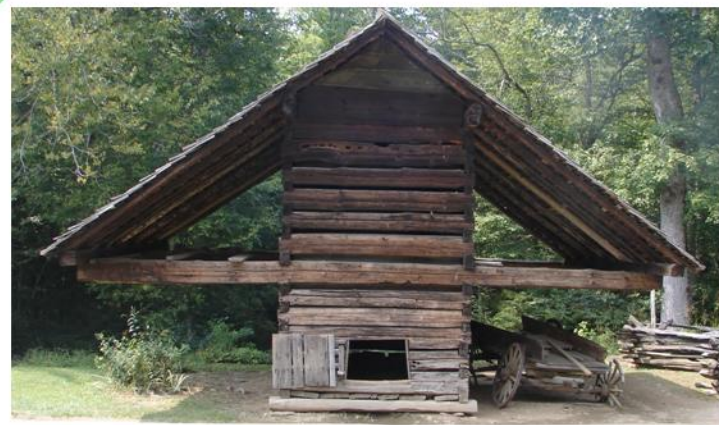
For all you vernacular architecture lovers: An unusual cantilever corn crib from the John Cable Mill Area of the Cades Cove Loop in the Great Smoky Mountains National Park. Note the wagon on the right. (K. O'Shea)
